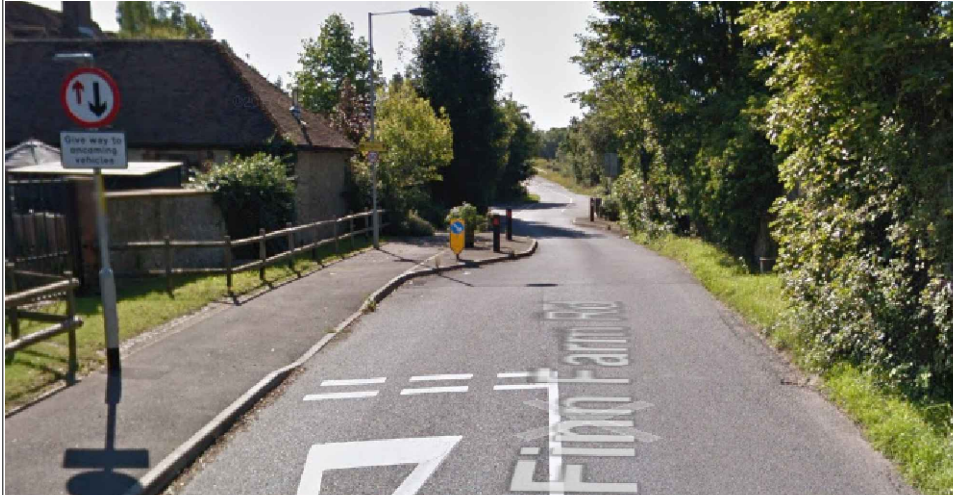
Example of Kerb Build out Traffic Scheme - Give Way Side. Finn Farm Road, Ashford
