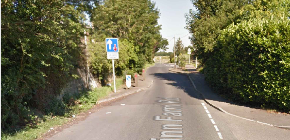
Example of Kerb Build out Traffic Scheme - Priority Side. Finn Farm Road, Ashford
