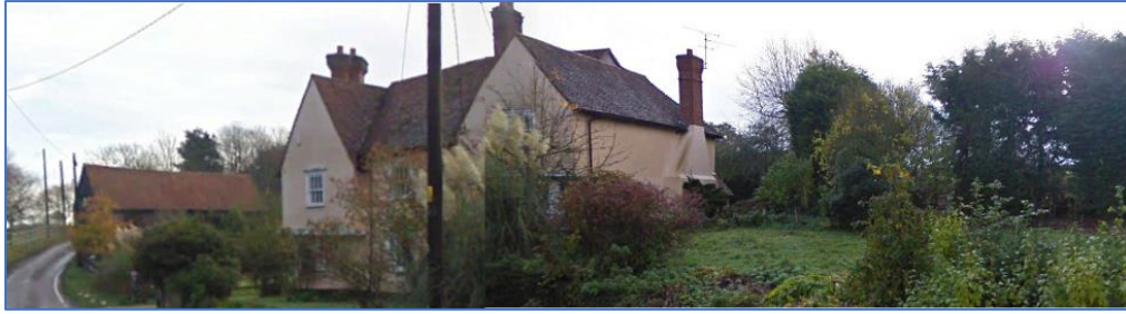
Figure 4 View of Goodman's Farmhouse from the lane, looking east, with listed barn beyond
