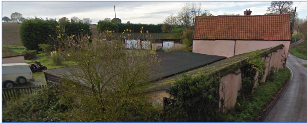
Figure 5 View of listed barn (pink render) looking towards PEA – not visible beyond conifer hedge
